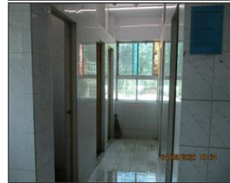
Photo of the sanitary facilities Inside Toilet.JPG
