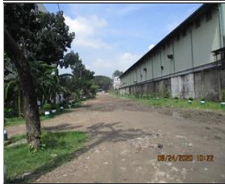
Photo of fire safety equipment Assembly Area.JPG
