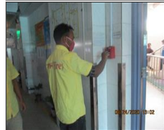
Photo of fire safety equipment Fire Alarm Test.JPG
